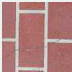
Cracking
